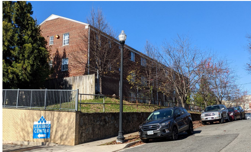
4. NORTH ODE ST. LOOKING NORTHWEST
