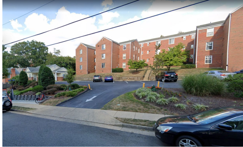
2. NORTH QUEEN ST. LOOKING EAST
